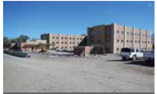
Bachelor Enlisted Quarters and mechanical HVAC building that provides heating and cooling to building.
