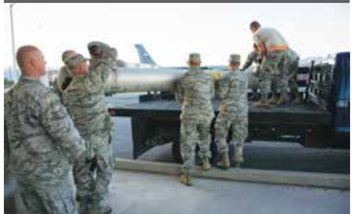
The 151st LRS Fuels Flight offloading a section of pipeline that is to be installed in its hydrant refueling system.
